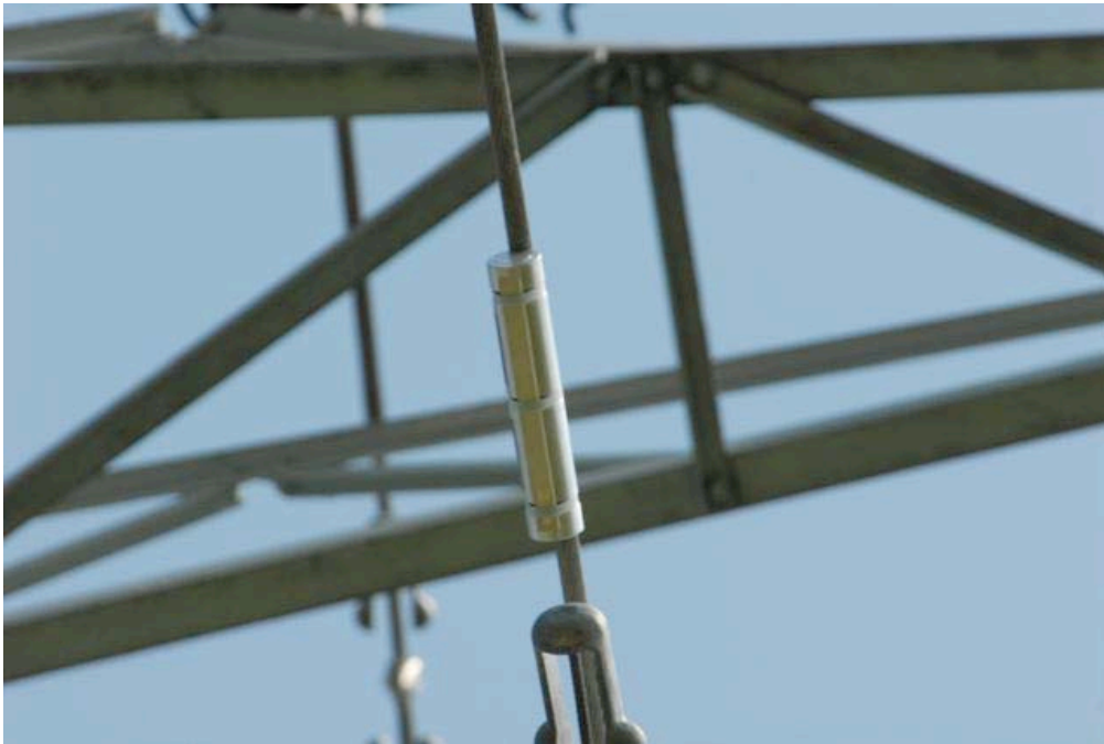
Pict. by courtesy of BEWAG Netz GmbH
